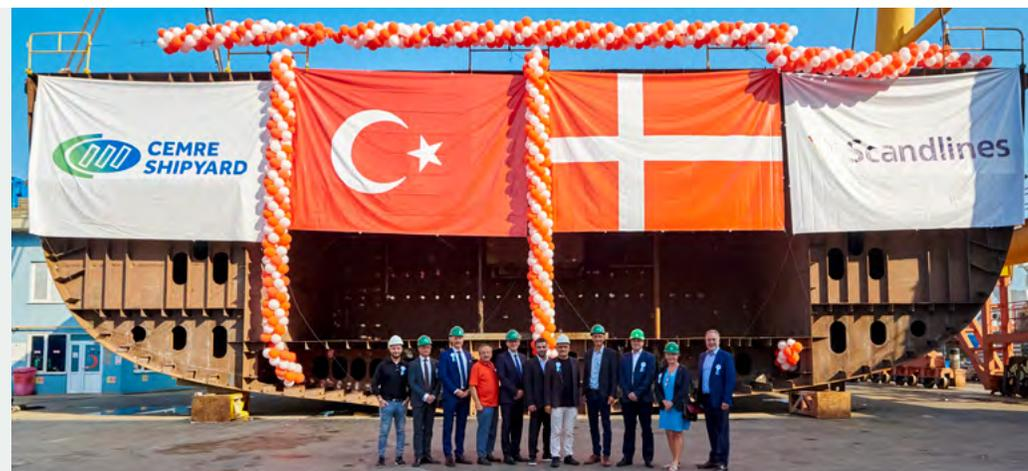
be built around one single keel but instead be comprised of 36 hull sections welded together to form the 9-deck ferry with capacity to transport 66 freight units and 140 passengers across the Fehmarn Belt in 70 minutes emission free and in 45 minutes as a hybrid ferry.
